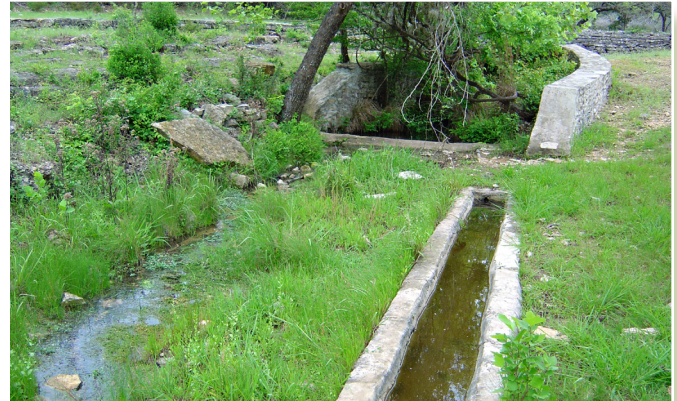
Protection around spring outlet with downstream watering trough for livestock Gillespie County (Photo courtesy of TPWD)
